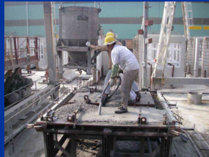
Concrete placement
