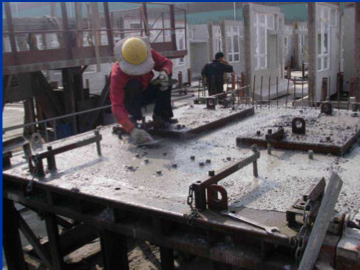
Trowelling concrete surface
